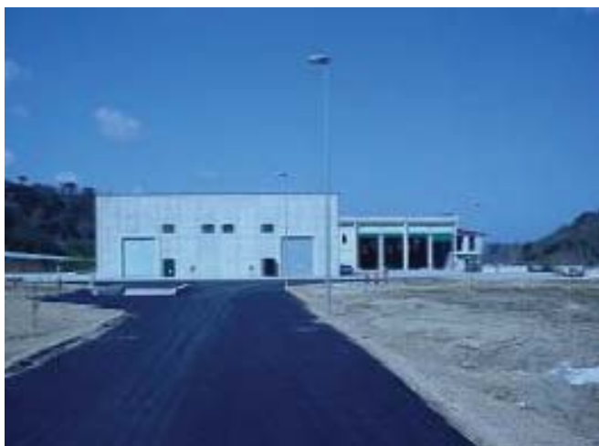
Plant at Vazzano, Southern Italy
